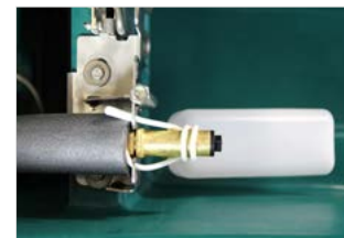
Option I : connected to water loop. Feed pipe is protected by a 24 V-20 W-2 m heating cable. 1 MAXIFLOW float valve + 1 heating element of 24 V-180 W
