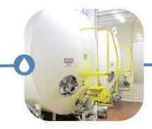
Cream from the separator is stored in these tanks. This cream will be part of the ingredients for most of the products made in the plant.
